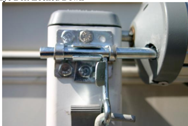
Eye Bolt Locked Down
